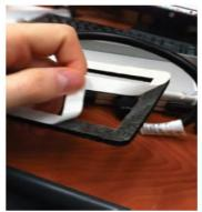
2. Feed the gasket over the cord and apply to back of face of the outlet. Press the gasket down onto the face until adhesive sticks.
