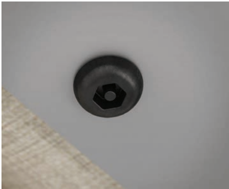
Tamper-proof fasteners are standard on all designs.
