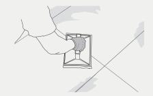
We recommend class CG2WA grout, as per EN 13888, specifically Butech Colorstuk Rapid. This coloured technical mortar is a grout for indoor or outdoor use. It sets quickly, is highly weather resistance and won't produce efflorescence.
