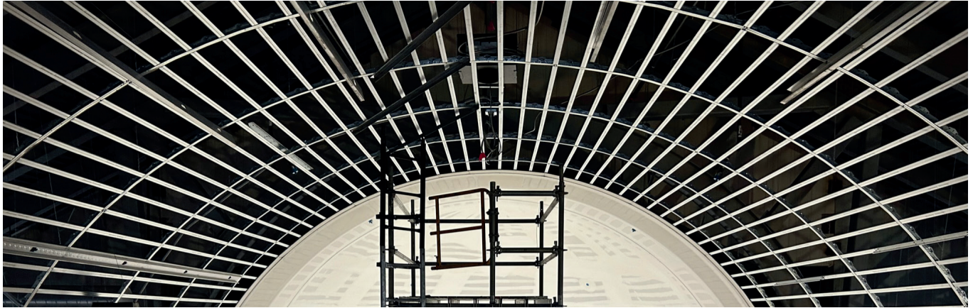
Faceted Drywall Grid System for curved drywall ceilings
