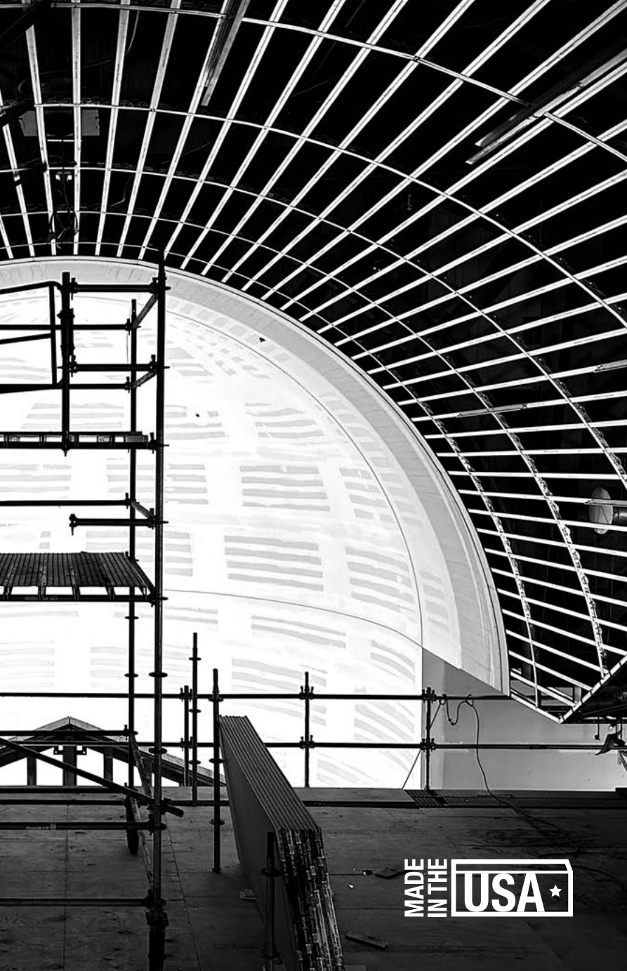
Flat Drywall Grid barrel vault installation
