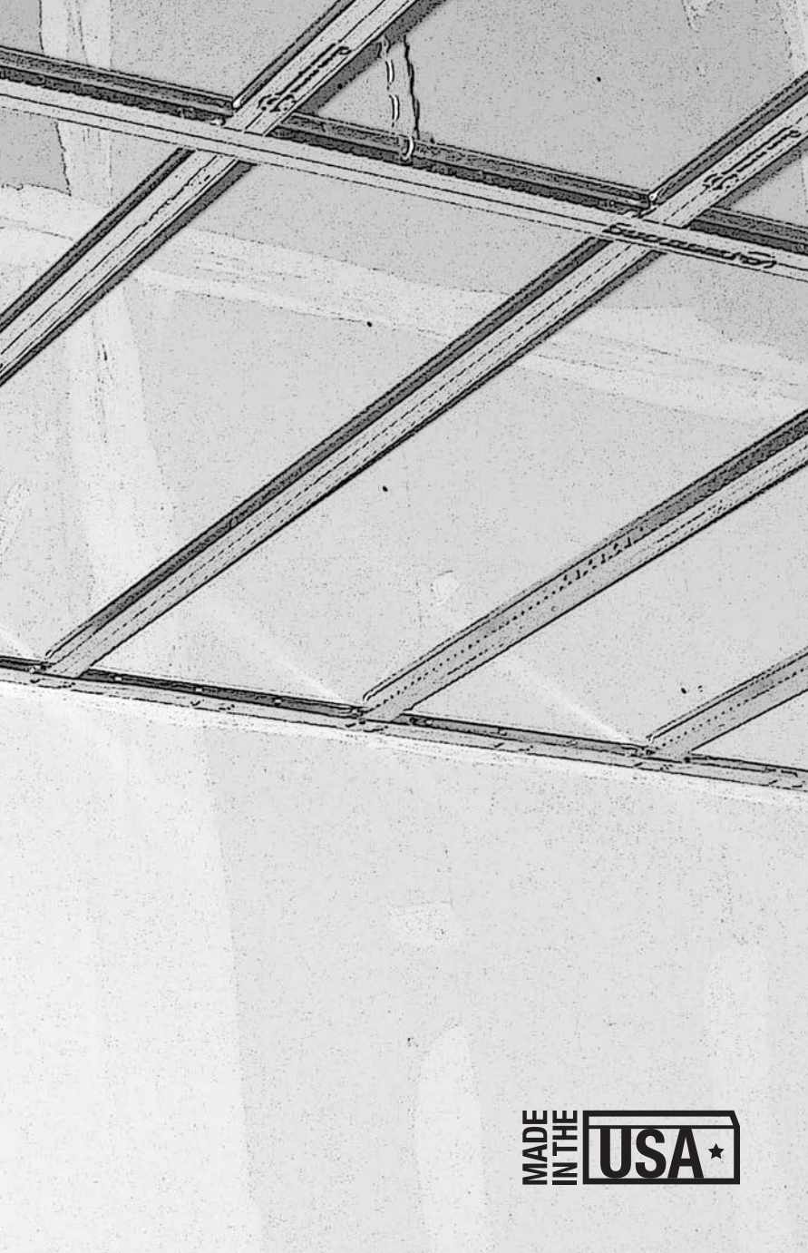
Flat Drywall Grid Installation
