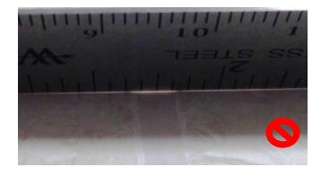
9. The finished seam will not show any wash and will be flush with both sides of the sheet vinyl.
