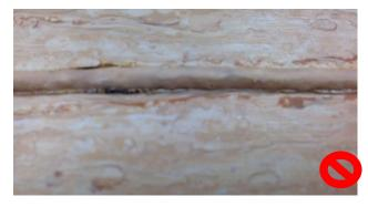
6. Weld gun temperature and operator speed are correct when the "wash" from the melted floorcovering and the weld rod is visible along both sides of the seam.
