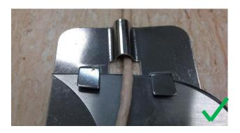
8. If the installer performs the final trim before the weld rod has been allowed to cool, the weld rod will become concave and the surface of the floorcovering can appear scratched. A concave seam will collect dirt when the floor is in use. Always allow the welded seam to cool for a minimum of 20 minutes prior to final trim.
