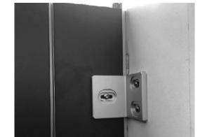
Pull the support leg down until it is firmly seated on the floor. Secure the support to the floor using two 6 mm plastic anchors and 4.8 mm x 38 mm screws. Pre-drill into the floor through the holes in the flange.
