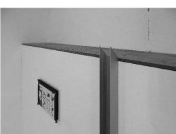
Adjust the remaining piece of the long U-bracket to the height of the system, and then attach the U-bracket, setting it perpendicular to the wall.
