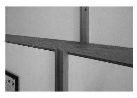
Adjust the short miter U-bracket, and then attach it to the shelf.
