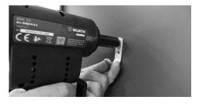
Pre-drill the hook mounting holes using a 4 mm drill bit. Only drill through the first wall of the door, not the entire door.
