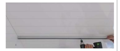
Attach ceiling brackets for the dividing panels and any outer walls (example, outerwall for a corner installation). The bracket for the dividing walls will be notched at the front. The dividing wall ceiling bracket needs to be cut onsite 15 mm shorter than the overall dimension. Cut the bracket on the non-notched side.
