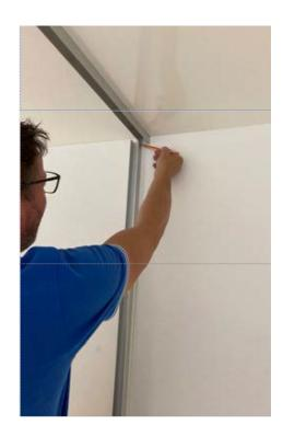
Mark the walls through the holes in the wall brackets. Using an 8 mm drill bit, drill at least 70 mm deep.
