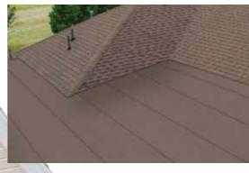
\* Waterproofing Underlayment is not typically applied at the eaves in climate areas not prone to snow and ice.
