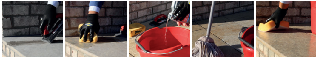
PIC 1. Fill joint with grout.
