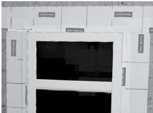
VYCOR® PRO Window Flashing
