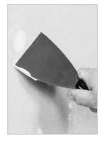
Larger breaks. Where the tape will not bridge the opening, use a keyhole or other saw to cut out an area around the hole. Cut the board back to the center of the stud on either side of the damaged area.
