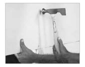
To install drywall horizontally (at right angle to the framing), start with the top board. Place together the tapered factory edge, moderately touching. Push the board firmly against the ceiling and fasten with nails or screws placed 7" from the interior ceiling angle. Space all nails 7" apart and screws 12" apart.
