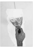
Torn face paper. Peel away any loose paper. Apply a very thin layer of joint compound, using a finishing knife large enough to cover the damaged area. Feather it to get a smooth finish. Let it dry for 24 hours and apply a second coat. if needed.
