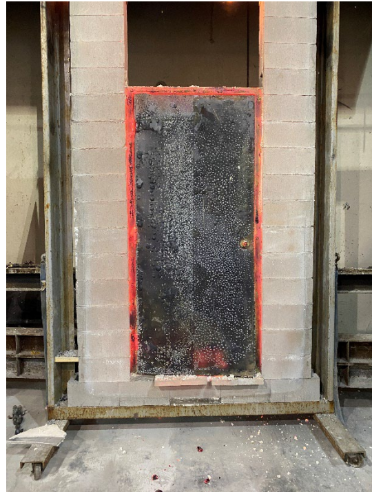
Figure 10: The exposed face of assembly 1 at the end of the fire test.
