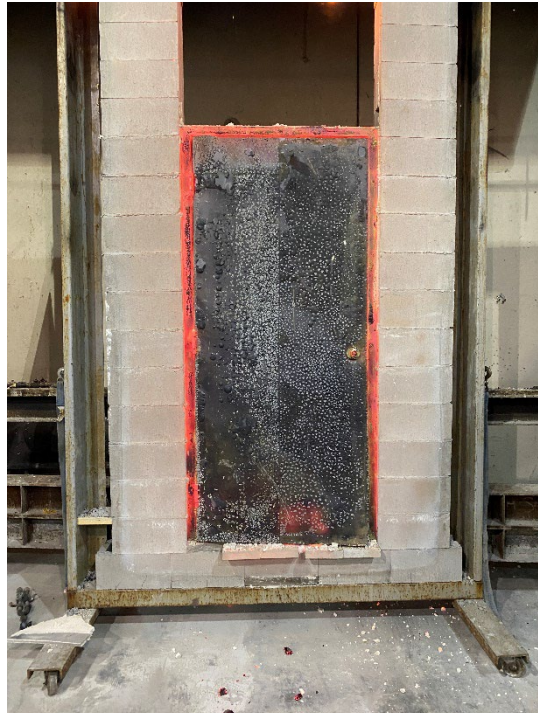
Figure 10: The exposed face of assembly 1 at the end of the fire test.
