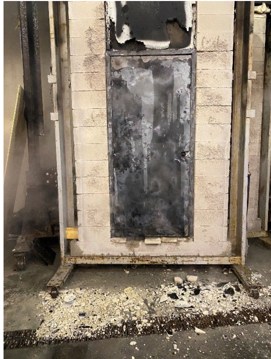
Figure 16: The exposed side of assembly 2 after the hose stream test.
