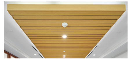
WoodWorks Linear Veneered Panels with perimeter trim
