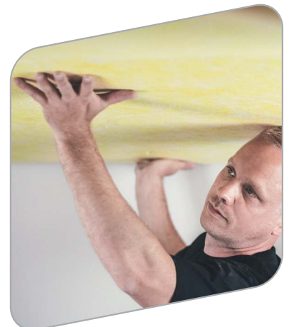
Installation glued with FADE Special Adhesive
