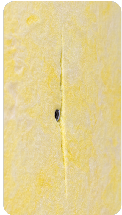
Recess the FADE Special Washer.
