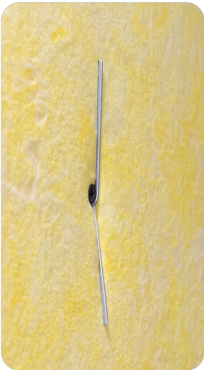
Screw the FADE Special Washer through the acoustic panel.
