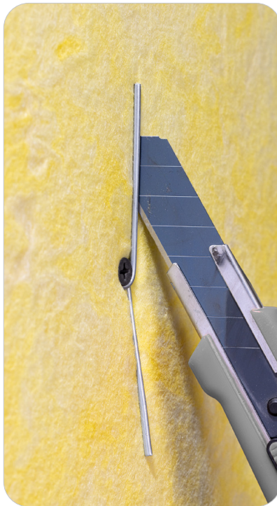
Make a slight incision on the side without the eyelet.
