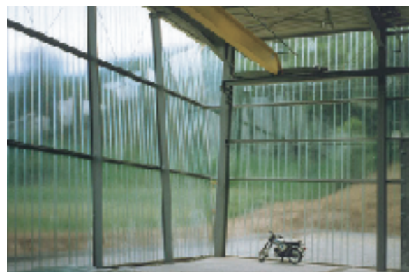
Industrial Hall, Germany
